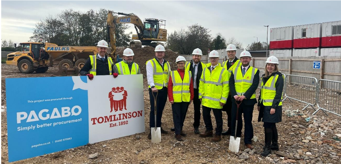
Pictured above: Construction beginning on the Air and Space Institute (ASI)
